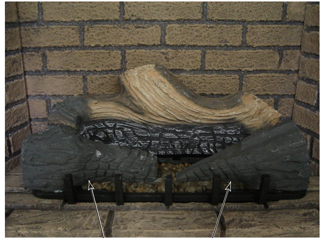
Left Front Log #5 — Right Front Log #3 Step 2 & 3 - Right (#4) and Left (#5) Front Log
