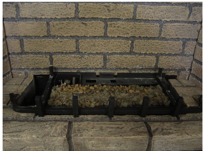
Figure 50 - Rock wool placement
